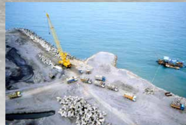
Border dike construction
