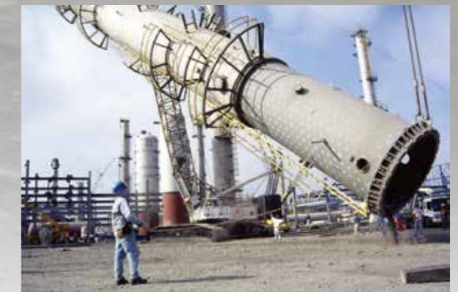
Plant and tower installation
