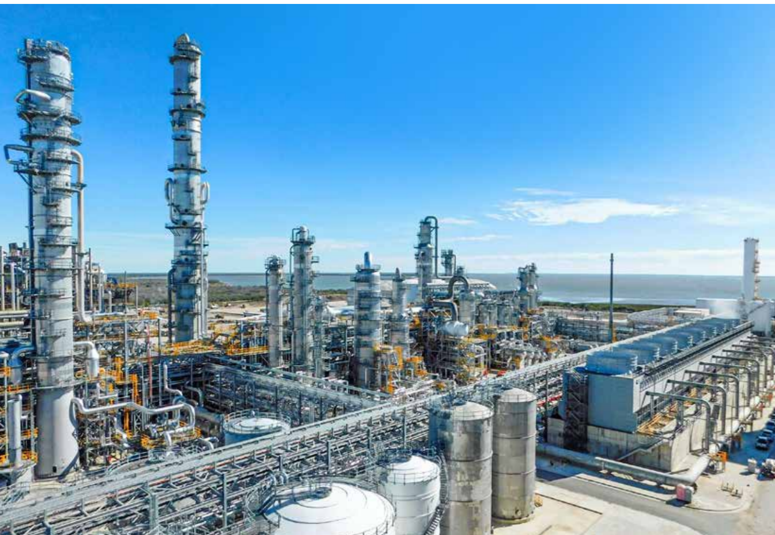
New Ethylene Glycol II plant in Point Comfort, TX
